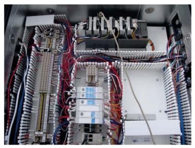
A FloBoss 107 being integrated with the Bear Failsafe System. The Bear FSC has a built in watchdog timer that can help detect an RTU failure, then independently shuts in the separator
