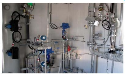
Two fast acting Bear SA linear actuators used on Fisher D2 dump valves and on the right a BA-15L being used for outlet back pressure control
